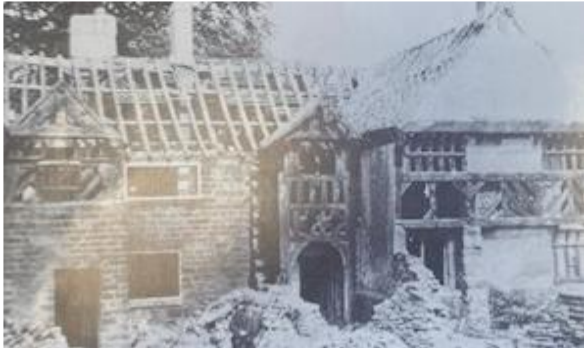
The demolition of the hall showed its Elizabethan timber frame.
