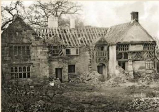
The Hall facing towards the South East in 1937 at the beginning of its demolition. The stone wing is believed to be the oldest part with the timber framing to the right perhaps dating from 1659. Courtesy of Barnsley Archives and Local Studies.
